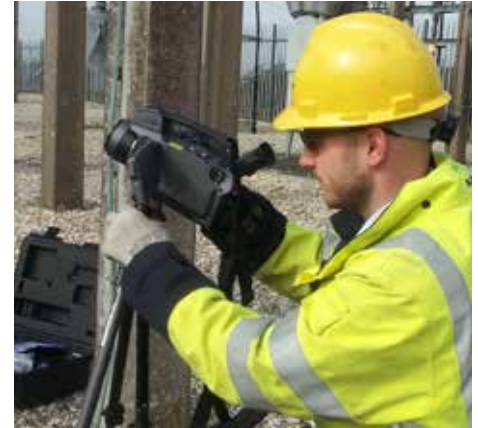
With the GF306, you can look at the switch gear equipment from a safe distance.
